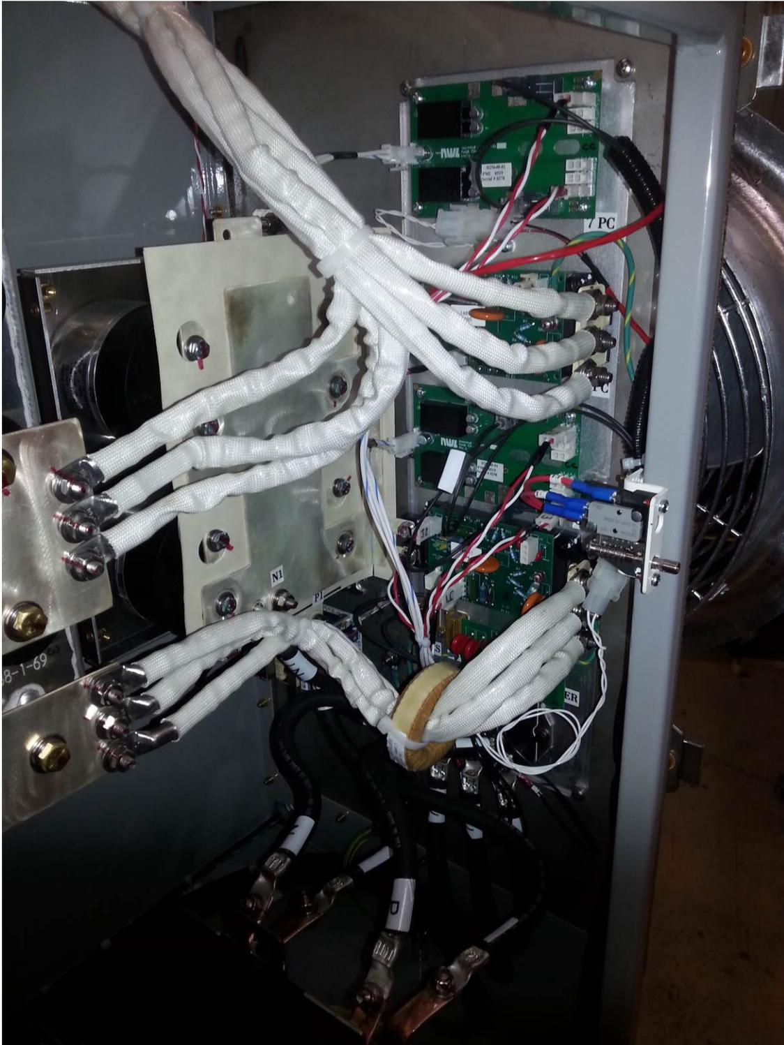
The layout of the heatsink will vary based on the kW rating of the unit. However, the method for the IGBT removal will remain the same.
